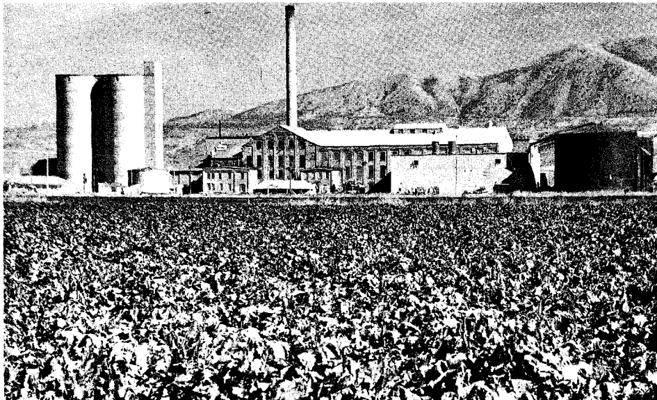
One of the oldest operating beet sugar factories in continuous operation in the United States. This U and I plant at Garland, nevertheless, utilizes many recent technological improvements.
